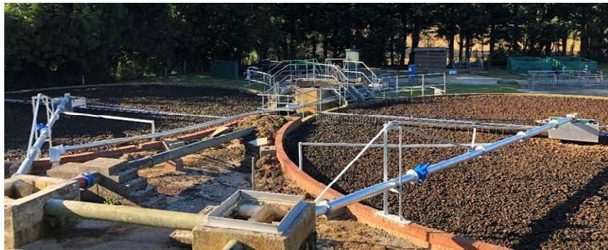
McGill Distributor installation at Iden WwTW
