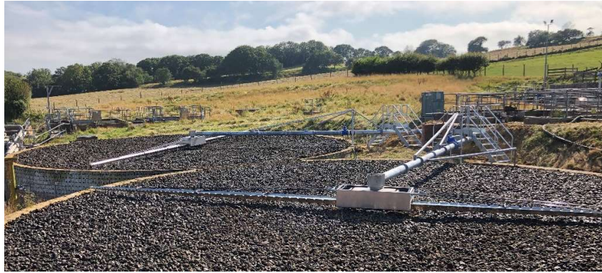
McGill Distributor installation at Fairlight WwTW
