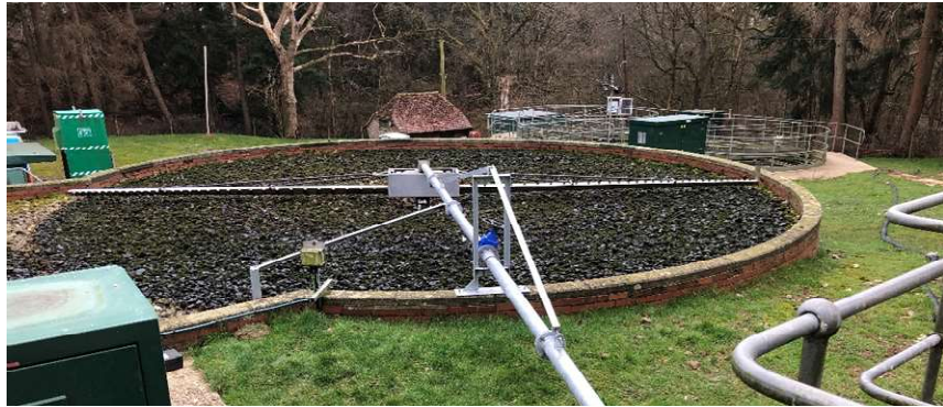
McGill Distributor installation at Handcross WwTW
