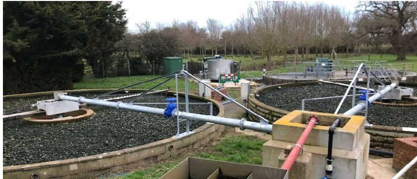
McGill Distributor installation at Appledore WwTW
