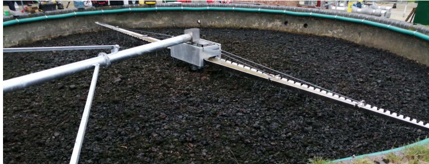
McGill Distributor installation at Plumpton WwTW
