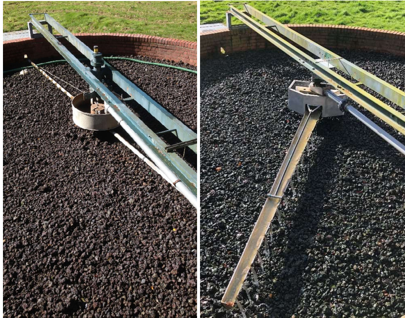
McGill Distributor installation at Itchingfield WwTW
